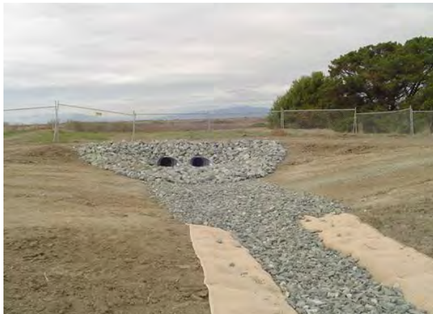
Concrete Rip-Rap Surface Water Drainage to Wetlands
