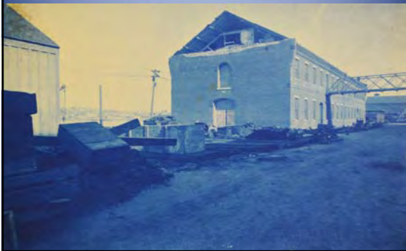
1898 Earthquake Damage at Mare Island
