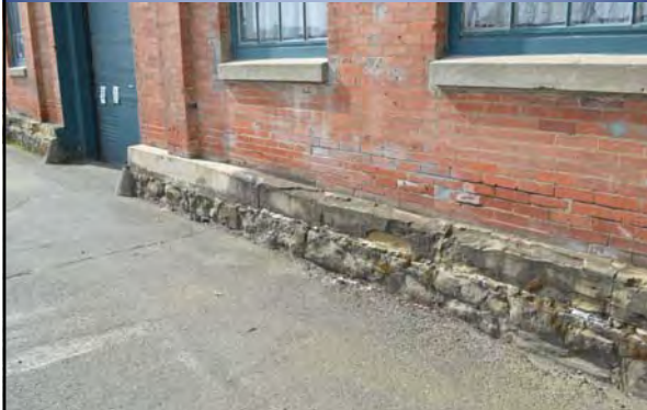
Stone Foundation of Bldg. 46, Stone was Quarried from Angel Island Sandstone
